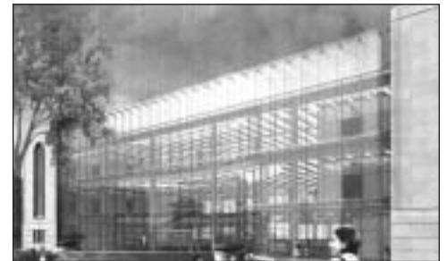
Front view of the handsome façade of Loyola University's Information Center. The facility, which looks out over Lake Michigan, will serve as a one-stop shopping experience in providing students with all types of information they need to do research.
