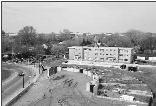
Foundation of the new 57-unit development, at Sheridan Road near Evanston.
